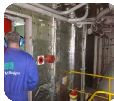
Insulation at Eng. Room Bulkhead, Emergency escape acceptable.
