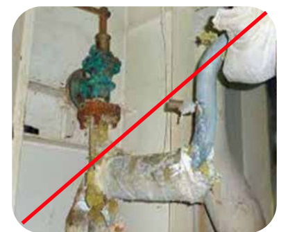
Emergency Fire Pump
